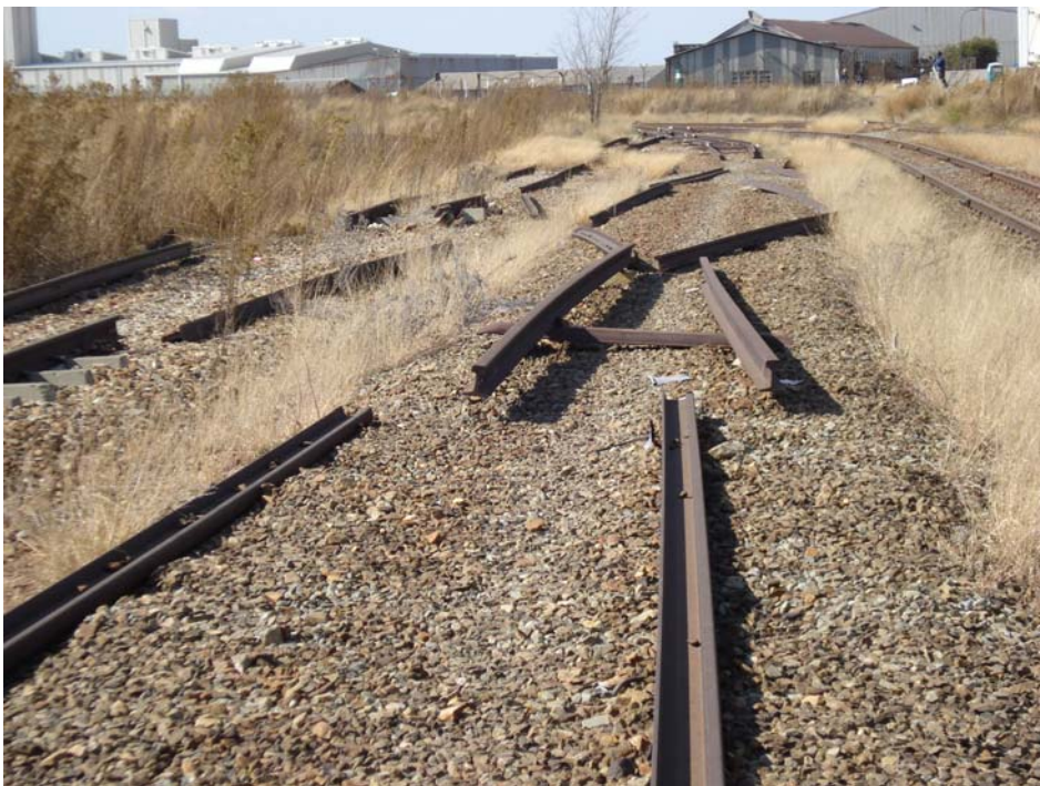
Railway lines in the Krugersdorp Industrial area
